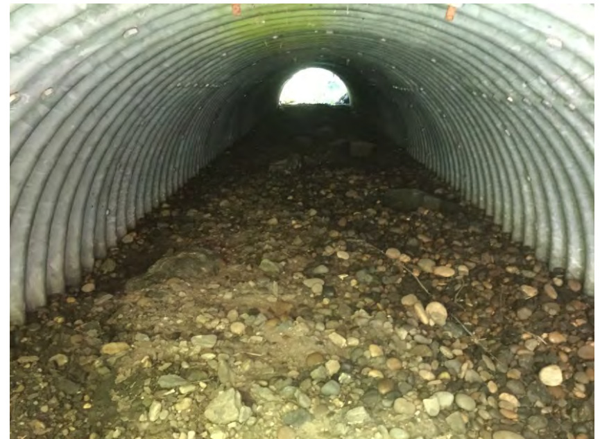
Looking through culvert from inlet
